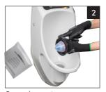
Spread armature grease onto the edge of the odor trap to make it seal tight against the urinal.
